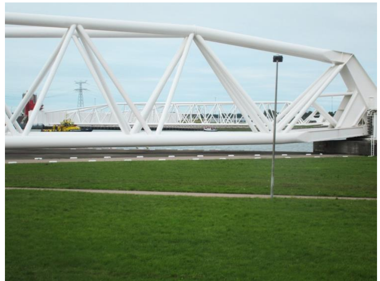
The Maeslant storm surge barrier is the most recent element of the Delta Works, completed in 1997. It is one of the three structures that protect the Port of Rotterdam. When it closes, the barrier's two massive doors fill with water. Within two hours, the doors sink to the bottom to hold back the flood waters. Photo: Kristen Grant
