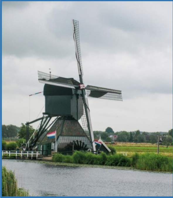
A windmill in the south of the Netherlands operates to pump water out of the floodplain and into the canal, creating drained land called a polder. Photo: Kyle Fritz
