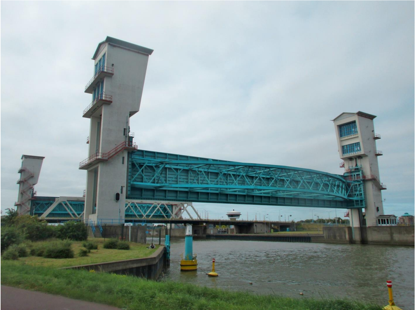
The Hollandsche IJssel storm surge barrier was the first component of the extensive system of Dutch flood protection measures called the Delta Works. The barrier was built in 1958, just five years after the devastating floods of 1953 that initiated the Dutch government's efforts to take full responsibility for flood protection in the country. Photo: Kristen Grant
