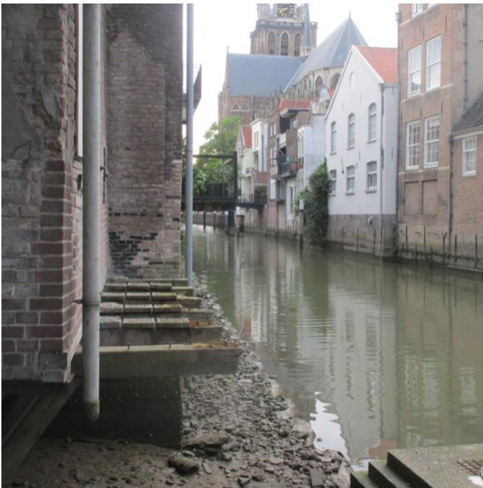
This area in Dordrecht in the Netherlands is among only a few populated locations in the country that is not protected by a primary dike, and therefore exposed to high risk of flooding from the ocean. Here visitors can see the bottom of the canal at low tide, an extremely rare sight in the Netherlands. Photo: Kristen Grant
