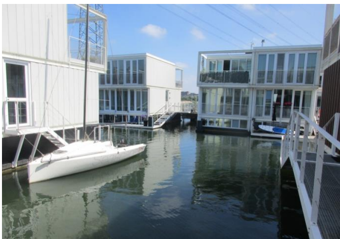
The floating neighborhood of IJburg in Amsterdam where homes are built over artificial islands raised from IJmeer Lake, as a means of food protection. Photo: Kristen Grant
