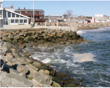
The Saco Bay seawall.
