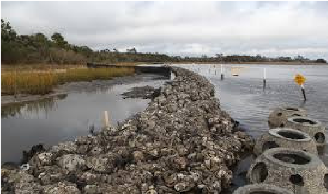
Artificial reef and reef-structures for erosion control and shellfish habitat are common in the Mid-Atlantic and Southern Coast.
