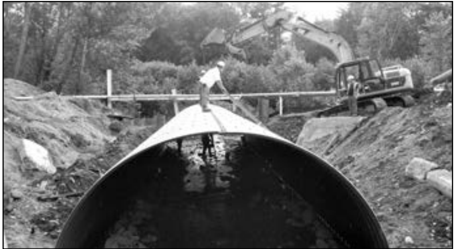
Crew installs larger pipe and culvert. (Submitted photo)
