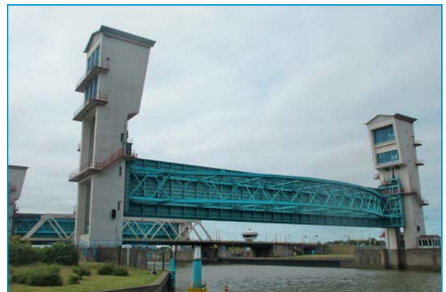
The Hollandsche IJssel storm surge barrier was the first component of the extensive system of Dutch flood protection measures called the Delta Works. The barrier was built in 1958, just five years after the devastating floods of 1953 that initiated the Dutch government's efforts to take full responsibility for flood protection in the country. Photo: Kristen Grant
