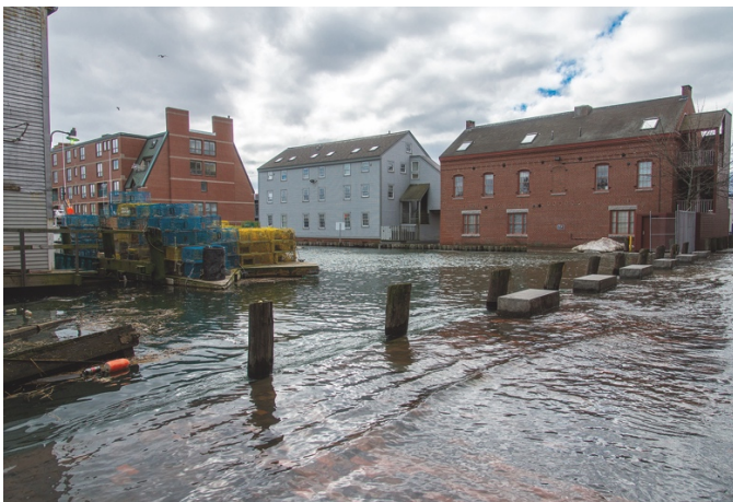
During the January 4, 2018 Nor'easter, powerful storm waves occurred at the same time as high tide. Water levels in Portland reached 13.8 feet, one of the three highest tides ever recorded. The tide remained above flood stage for nearly three hours, causing millions of dollars in damage statewide (Schmitt and Uteuova 2018). Photo: Corey Templeton licensed under CC BY-NC-ND 2.0
