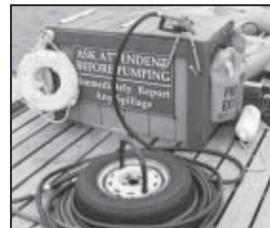
At Paul's Marina in Brunswick, the fuel nozzle is returned to a box where it drips onto absorbent pads—helping to prevent any fuel from reaching the water.
