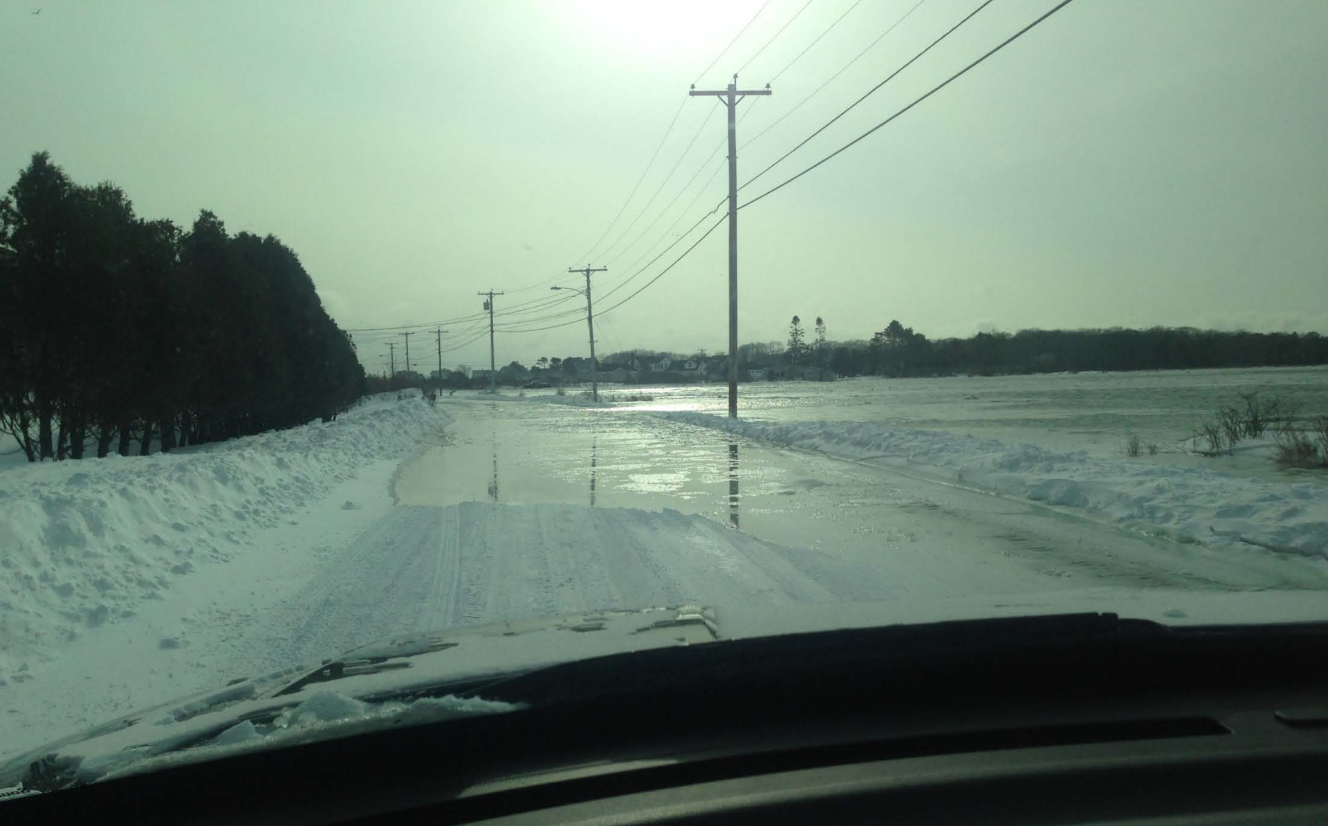
This is our “new” coastal inundation “hot spot” on Granite Point Road as reported by Biddeford EMA Roby Fecteau in Real-time during the storm
