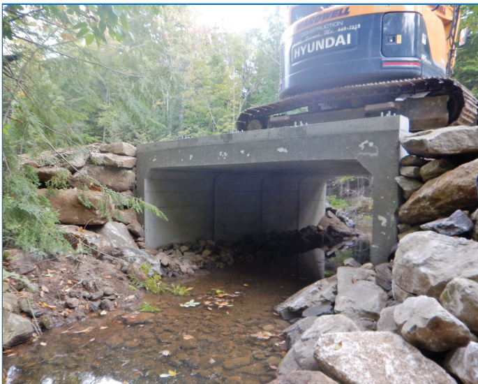
Winkumpagh Brook before ▲ and after ▼ Stream Smart road crossing
