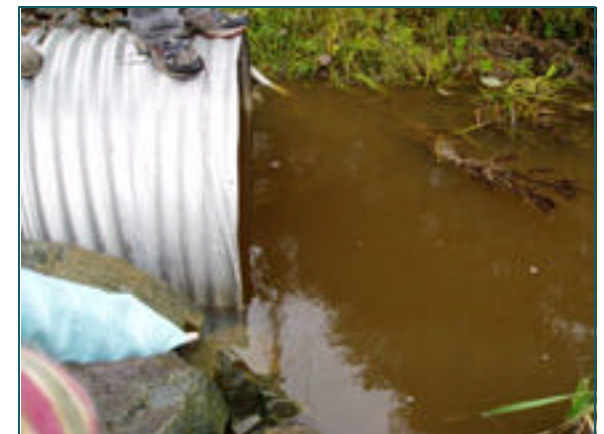
Northeast Creek culvert.
